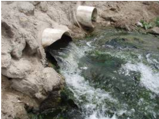
Pipe discharge at site
