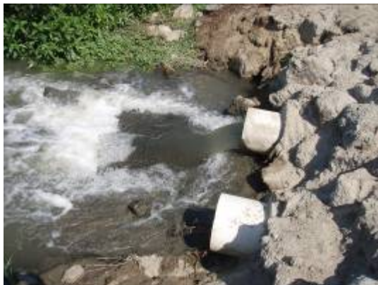
Pipe Discharge at site
