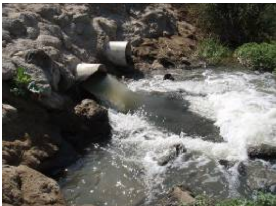
Pipe Discharge at site
